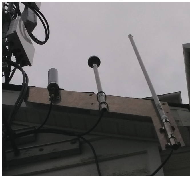
Illustration 3: Three small ancillary antennas are required for communications and time-synchronization.
