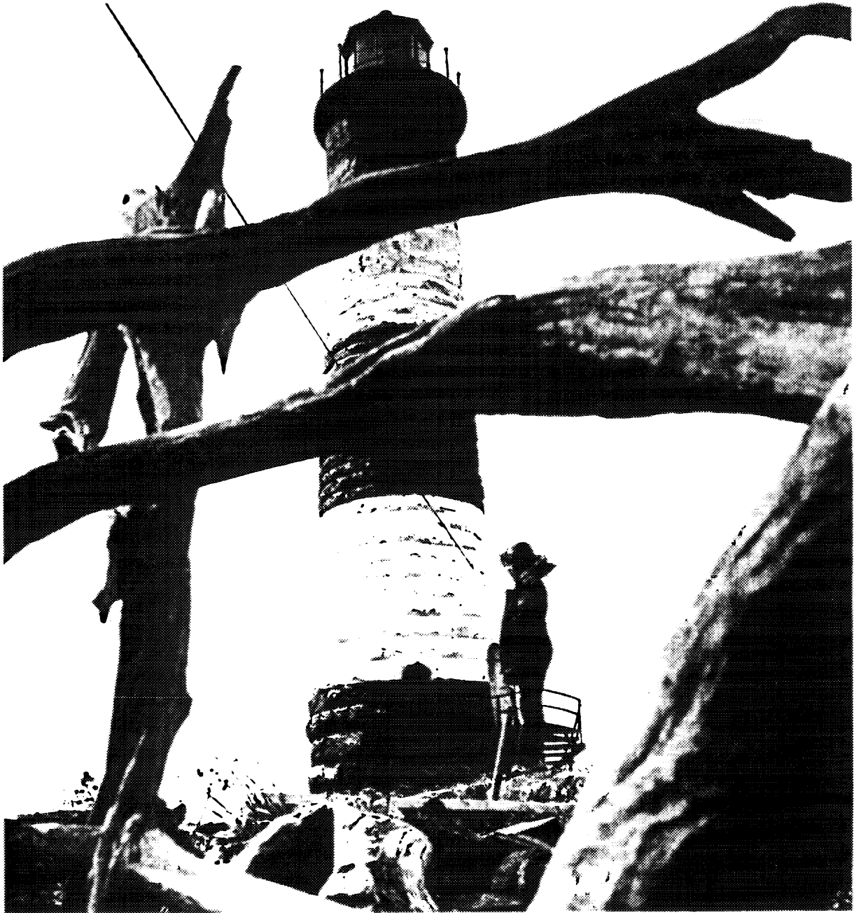
8 Race Rocks Lightstation, a more recent view. (Donald Graham, Keepers of the Light: A History of British Columbia's Lighthouses and their Keepers (Madeira Park, B.C.: Harbour Publishing, [1987], p. 32.
