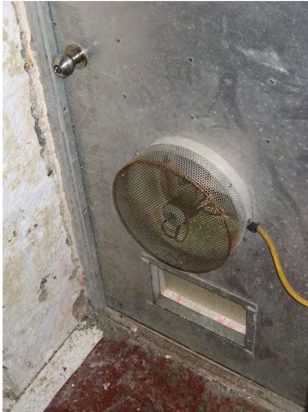
Figure 48: Ventilator set into the entrance door. (HCN/2007)
