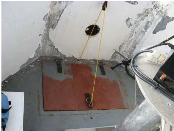
Figure 44: Access hatch to the lantern. (HCN/2007)
