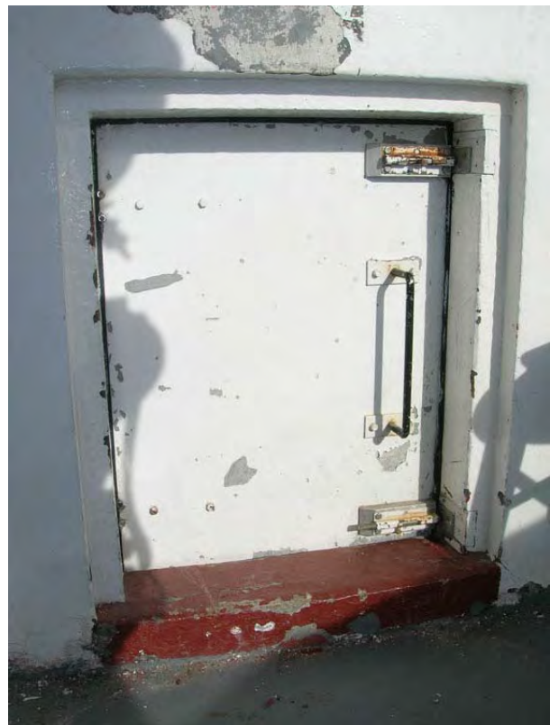
Figure 43: Lantern door to gallery. (HCN/2007)
