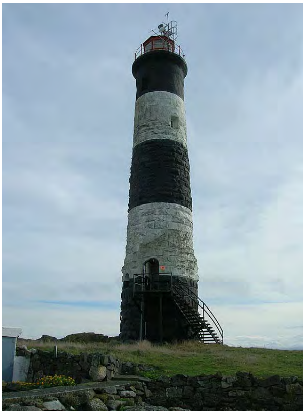
Figure 8: West view of the tower. (HCN/2007)
