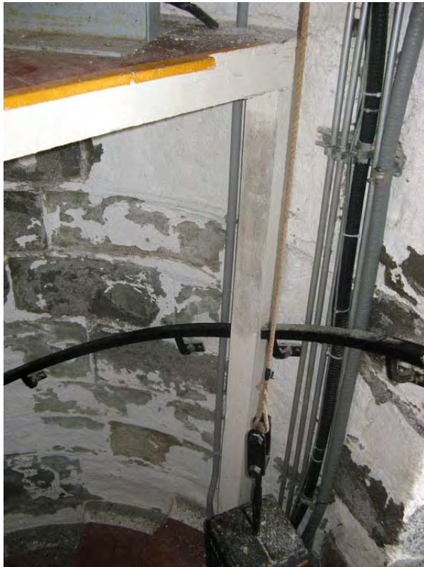
Figure 30: Post supporting the wood platform. (HCN/2007)
