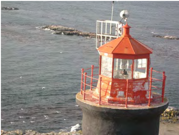
Figure 32: Exterior view of the lantern. (HCN/2007)
