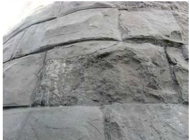
Figure 13: Natural stone and formed cement parging at the foundation level. (HCN/2007)
