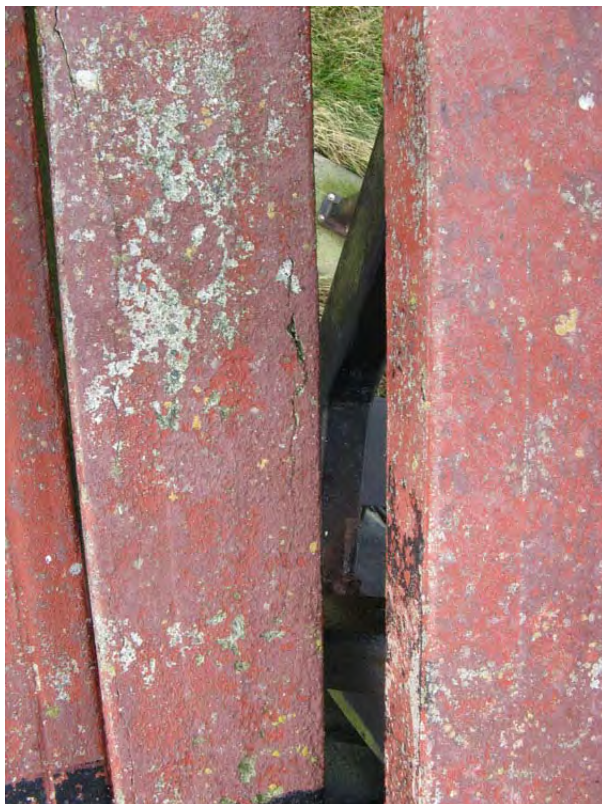
Figure 58: Cracked concrete treads. (HCN/2007)
