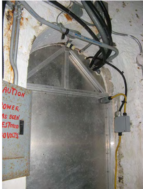
Figure 55: Interior view of the door transom and wiring entry. (HCN/2007)
