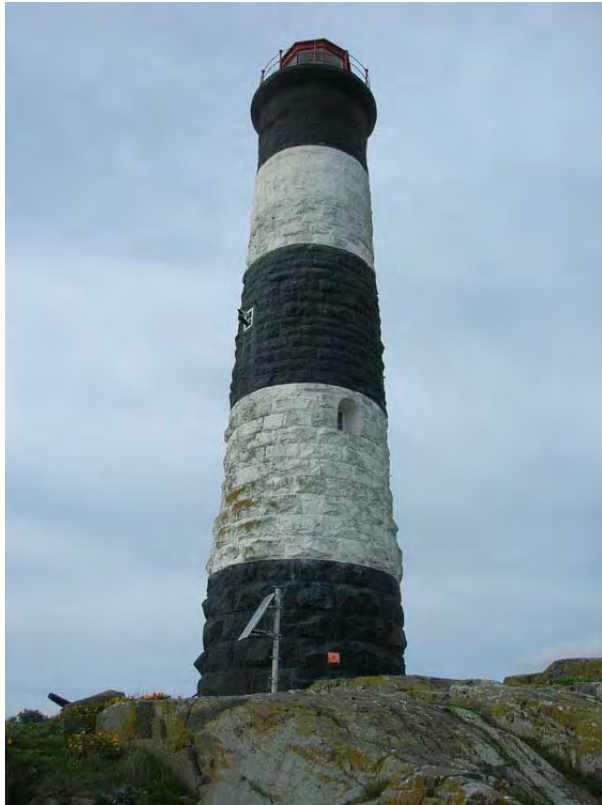
Figure 10: East view of the tower. (HCN/2007)
