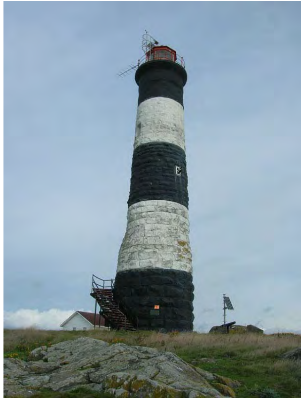
Figure 11: South view of the tower. (HCN/2007)
