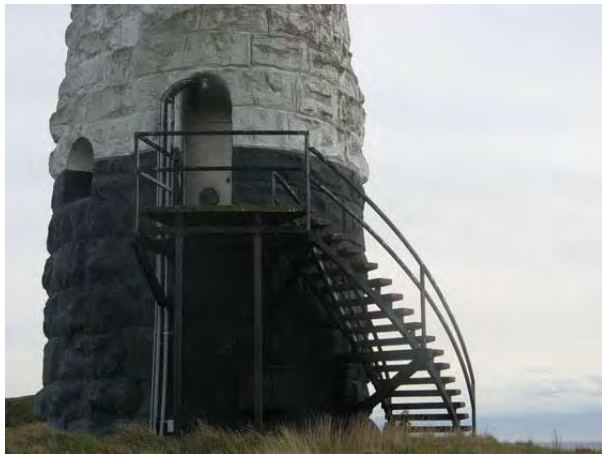
Figure 56: The exterior stair leading to the tower door. (HCN/2007)
