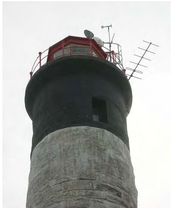
Figure 17: “Guniting” wall surfaces in the top third of the tower. (HCN/2007)
