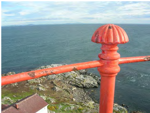
Figure 46: Guardrail post and decorative ribbed head. (HCN/2007)
