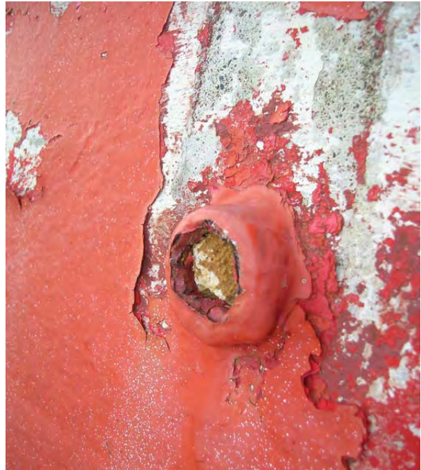
Figure 41: Plugged exterior condensation gutter drain. (HCN/2007)
