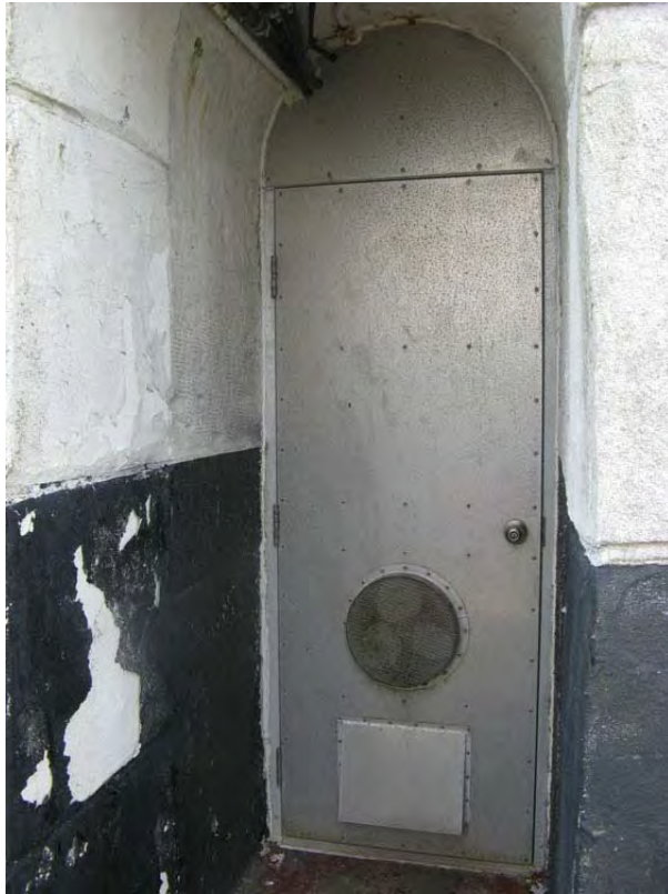
Figure 54: Exterior view of the door. (HCN/2007)
